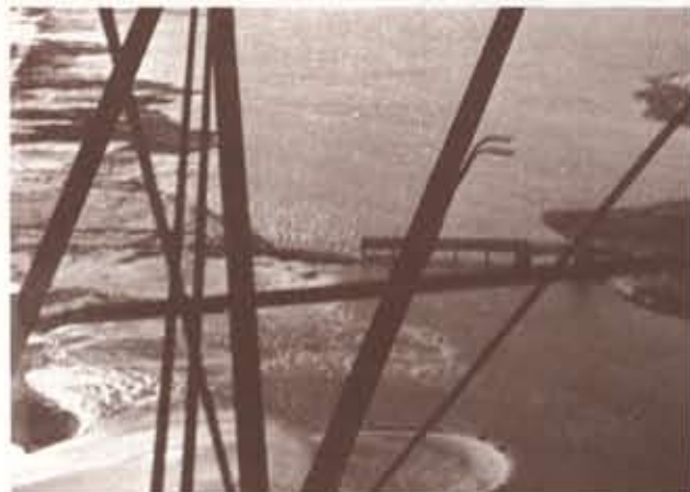
West Bay Bridge in Westhampton Beach showing the total destruction of the south approach. This photo (and the bottom photo) was taken from a plane the day after the hurricane by Thomas J. White and Stephen F. Griffing, Jr.
