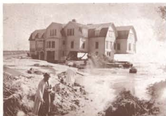
The E. M. Byers house seems to be floating on air, and very nearly was, with much of its foundation washed away. (Corcoran)
