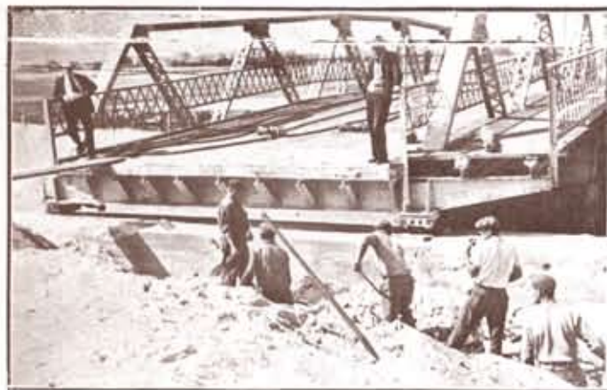
Reconstruction, Quogue Bridge
