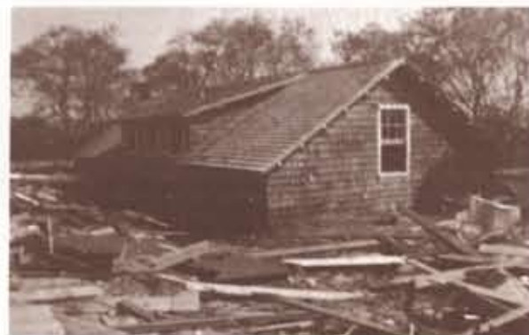
The top of this garage had been made into a playroom. When the waters subsided, the wreckage settled some distance away, bottom of the building vanished, and ping pong paddles still lying on the table.
